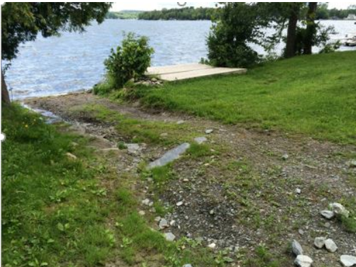
Eroding path leading to lakeshore
